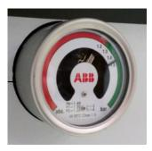
Displays the gas pressure and provides an analog indication of the value. The information can be seen on the front of the panel and can also be transmitted to another location by means of wiring and a terminal box. See circuit diagram.
