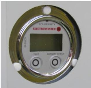
Monitors the gas pressure and provides an alarm if the pressure drops too low.
